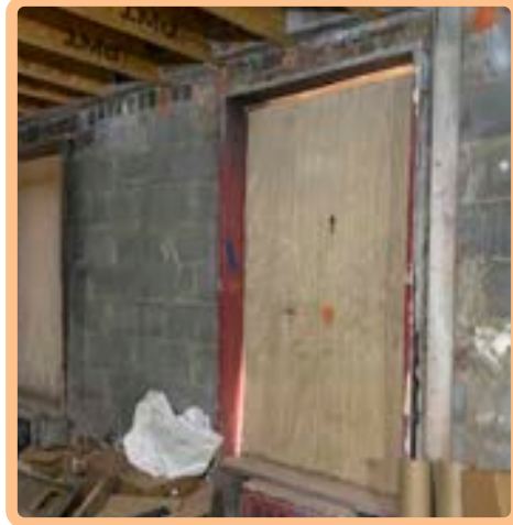
02: Window opening for new
