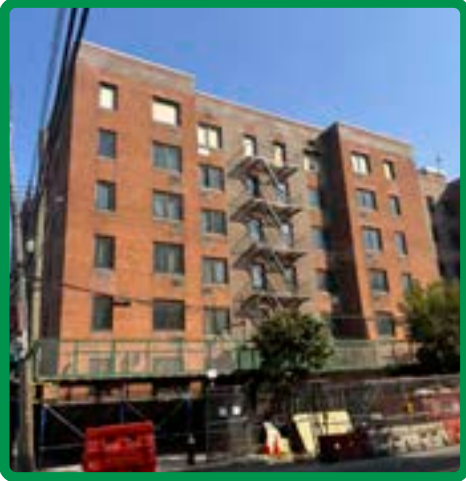
01: Building facade from Watson Ave
