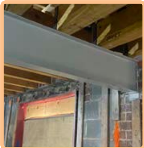
04: New structural steel transfer beam
