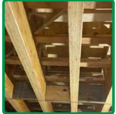
03: Reframed roof with wood structure
