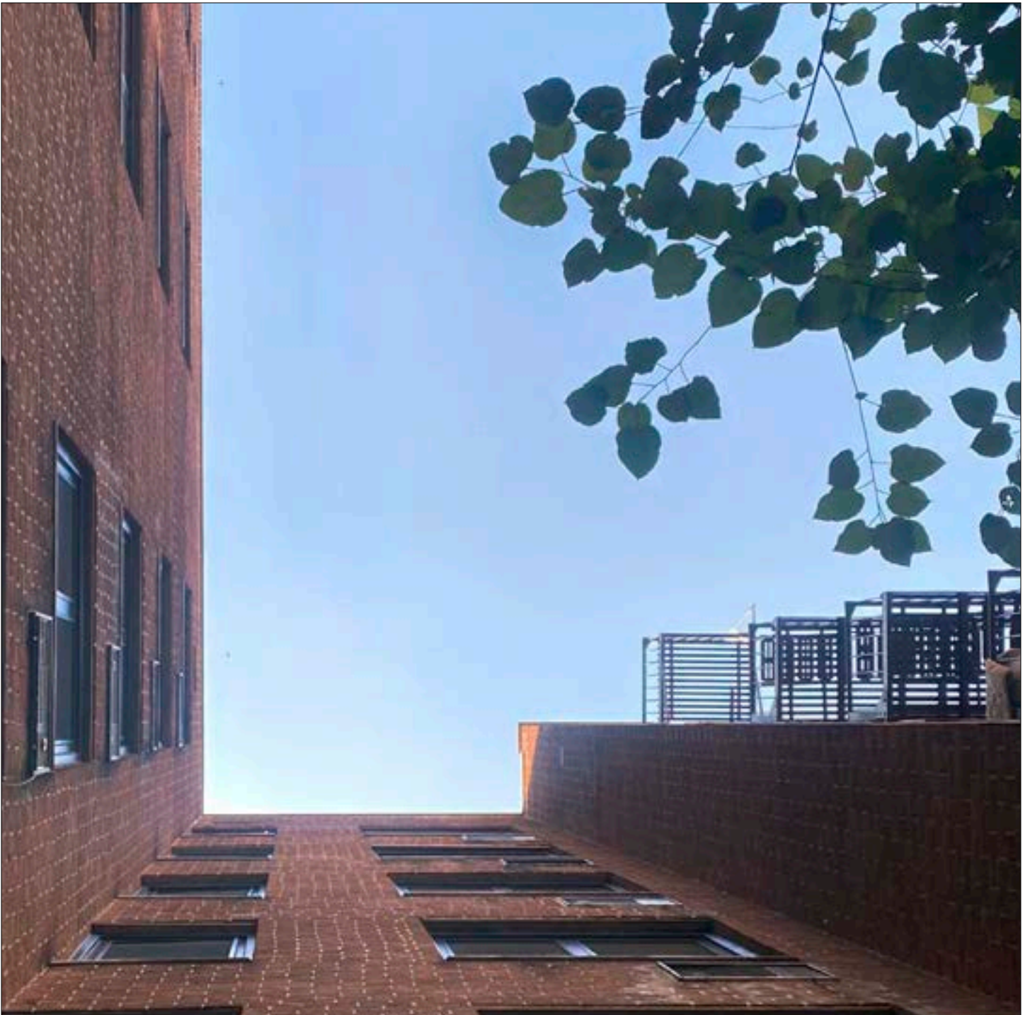
VIEW OF WATSON BACKYARD FACADE
