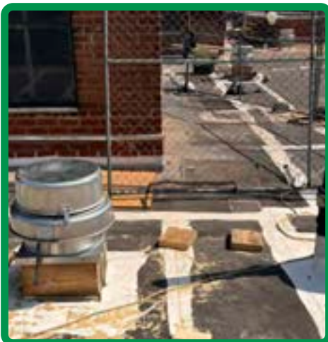
07: Cleaned rooftop fan
