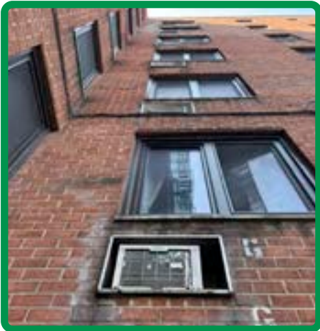
04: Ill fitting window AC unit; creates thermal break
