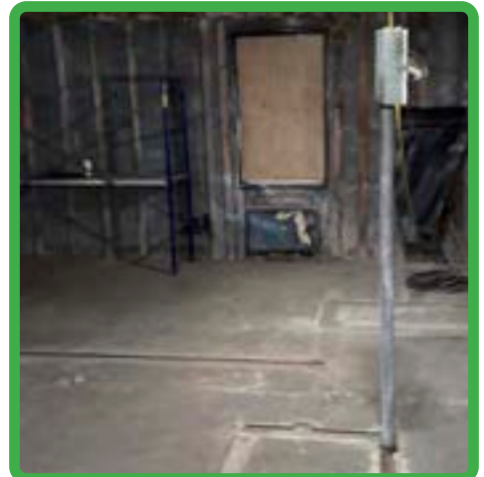
06: Wood sheathing floor
