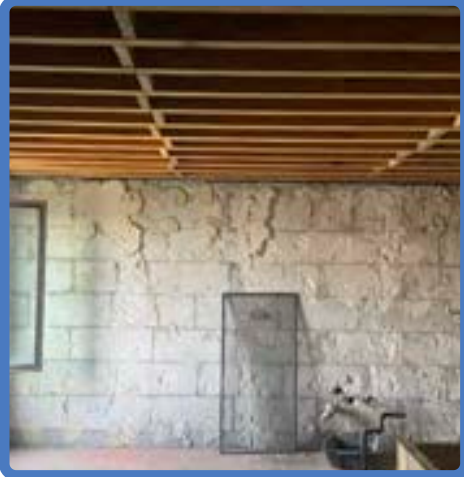
01: CMU party wall between apartments
