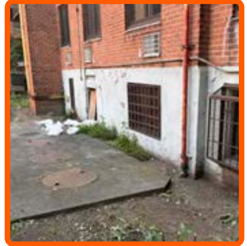
03: Concrete pad for oil tank
